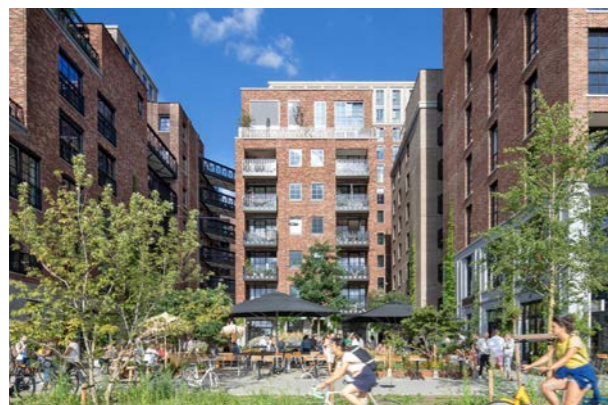
Coolhaven in Rotterdam, door Little C.
